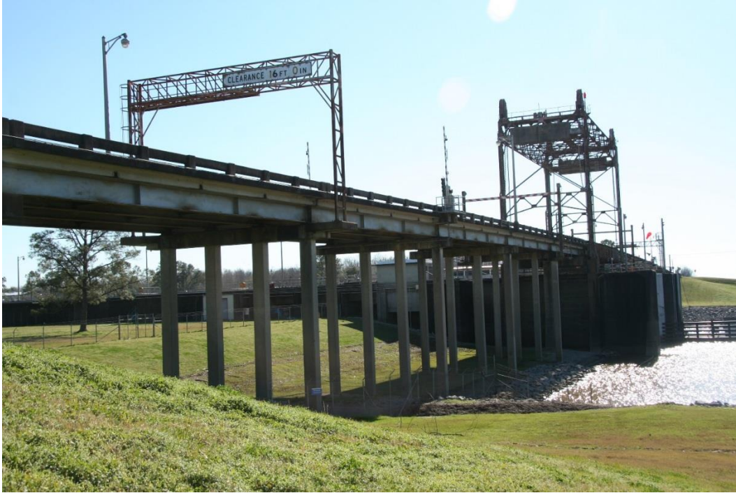
Condition Photo 8: North approach spans, looking east.
