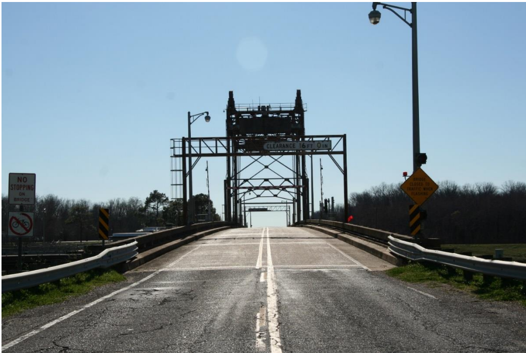
Condition Photo 9: North approach to bridge, looking south over north approach spans.
