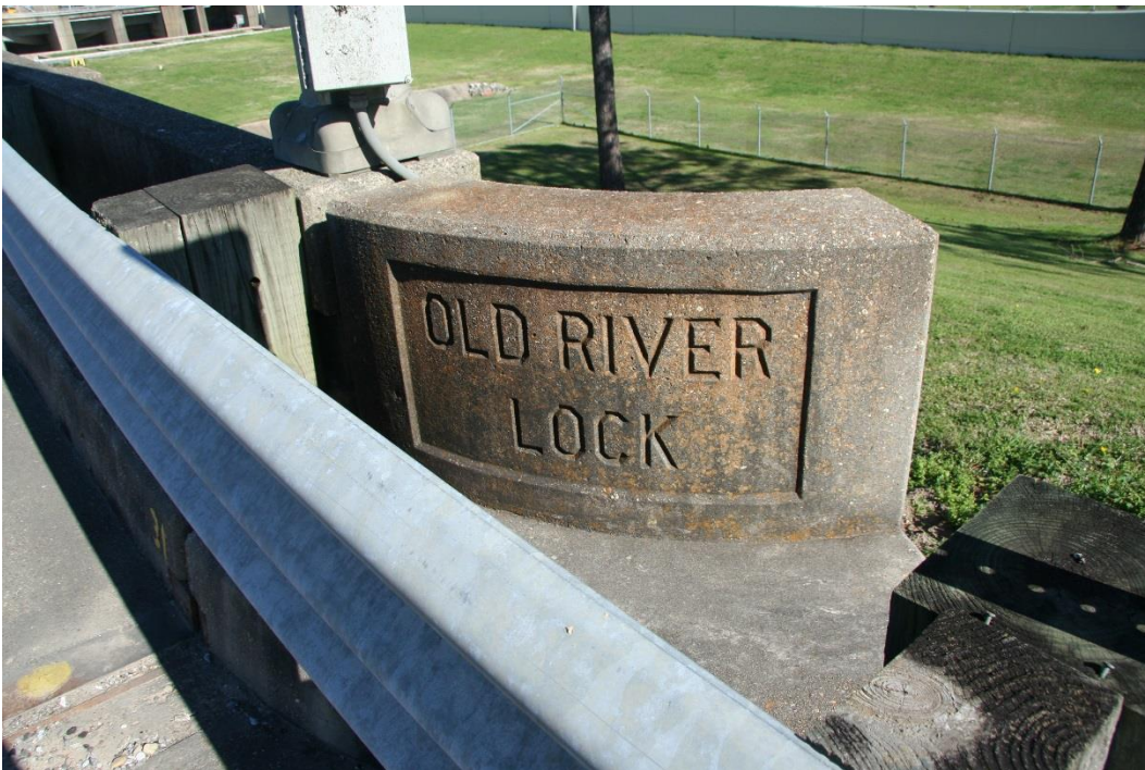
Historic Fabric Photo 2: Endposts on concrete railing of approach spans.
