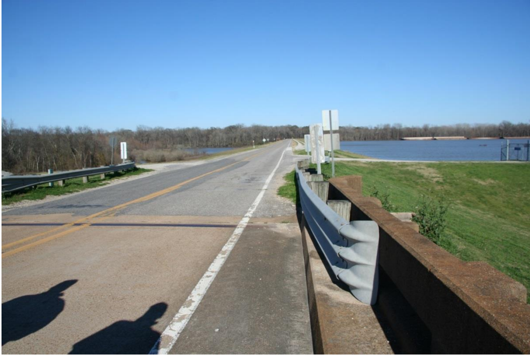
Condition Photo 4: North approach top bridge, looking north.
