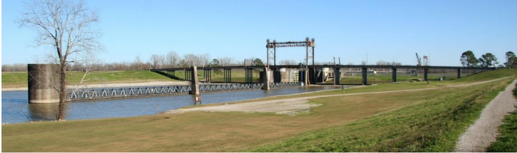
Condition Photo 16: Overview of approach to lock and bridge, looking southeast.
