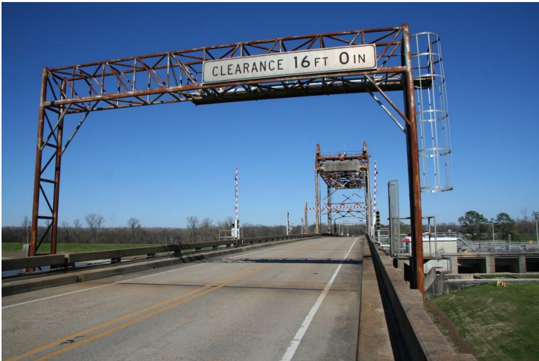
Condition Photo 3: South overhead clearance sign; south approach spans.
