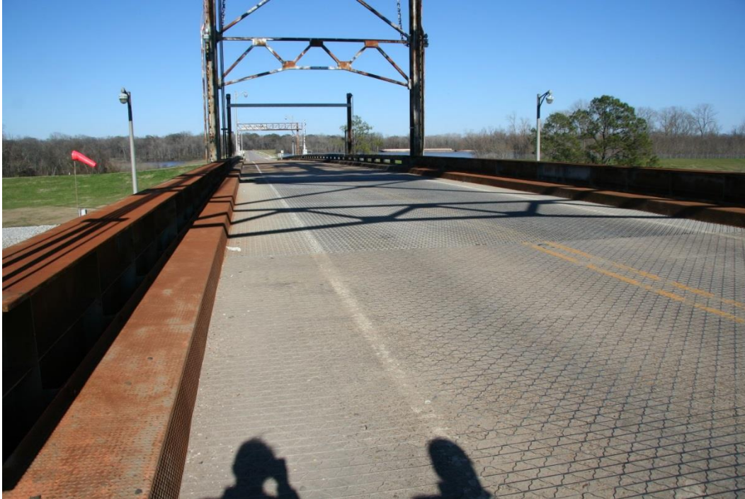
Condition Photo 14: Lift span deck and walkway, looking north.
