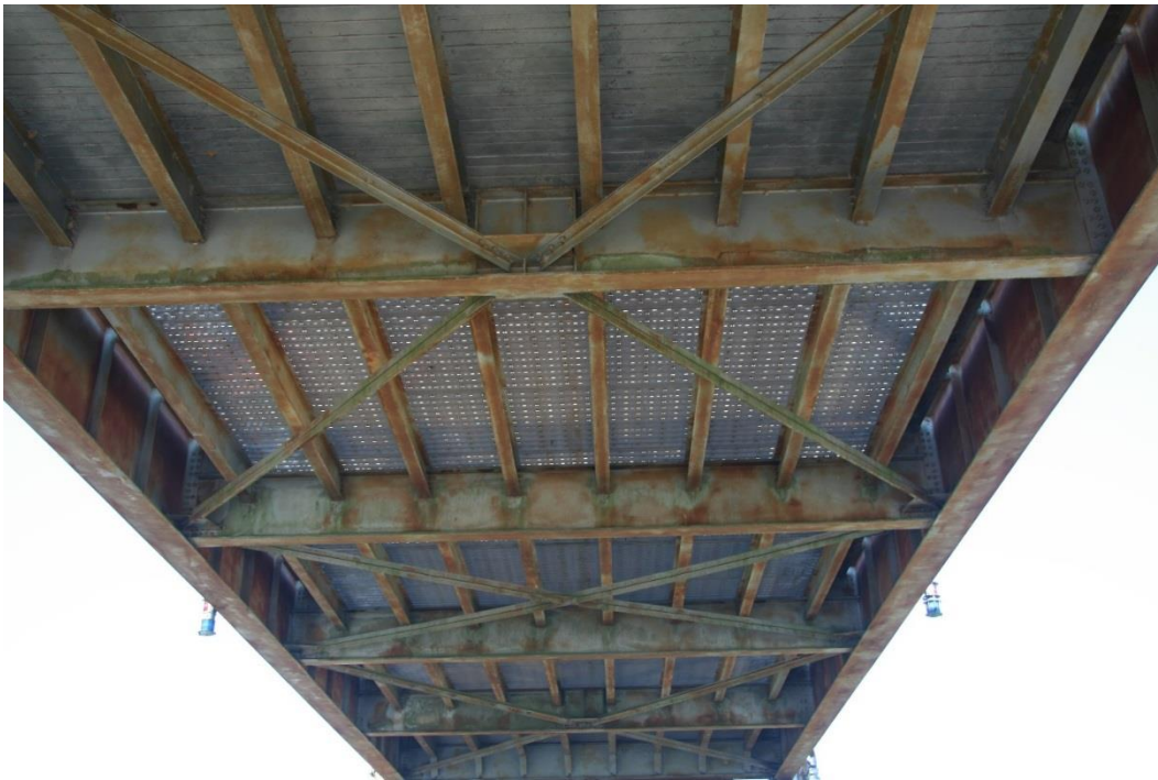
Condition Photo 15: Underside of lift span showing steel framing and deck.
