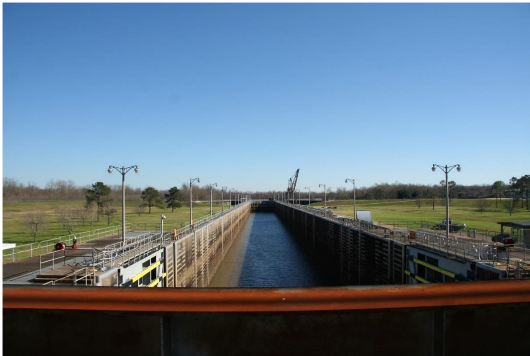
Condition Photo 11: Looking southeast at lock and dam.
