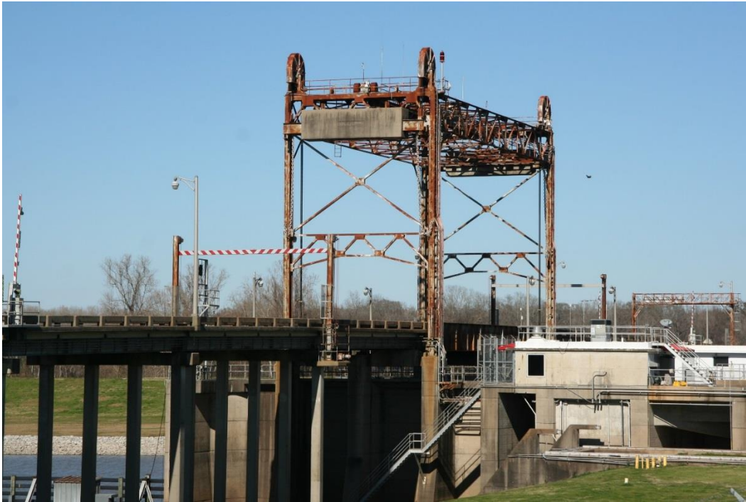
Condition Photo 1: General view of south side of bridge and operator's house, looking north.
