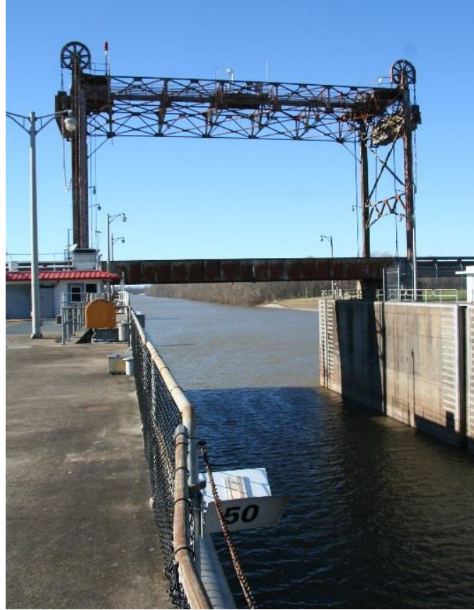
Character-defining Feature Photo 3: Design and construction of a bridge over a navigation canal.
