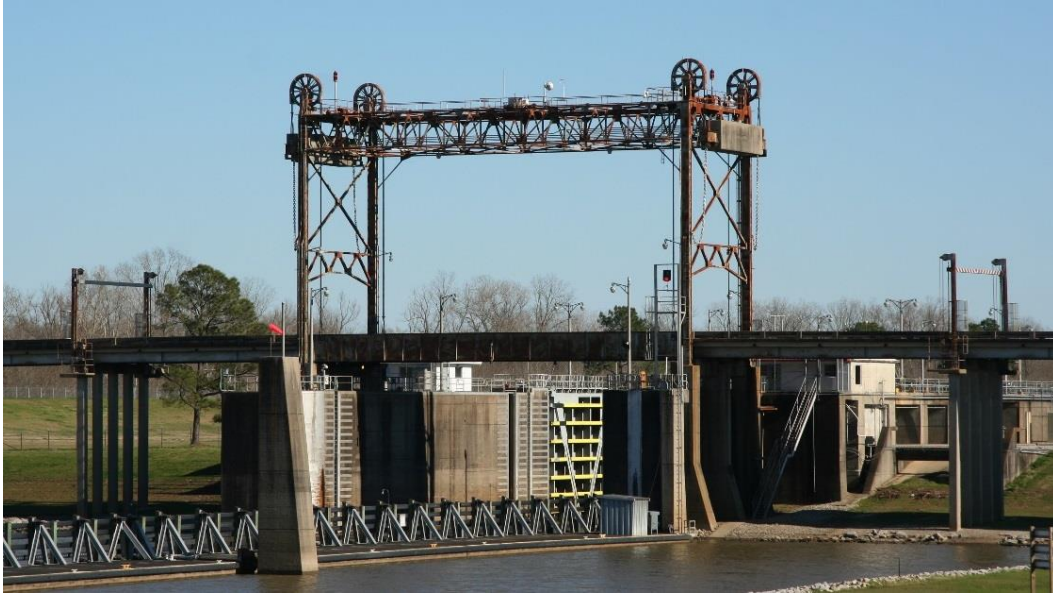
Character-defining Feature Photo 1: Design and construction of a vertical lift span with central drive machinery. The operating machinery, located at the center of a platform, drives the four sheaves on each corner of the lift towers.
