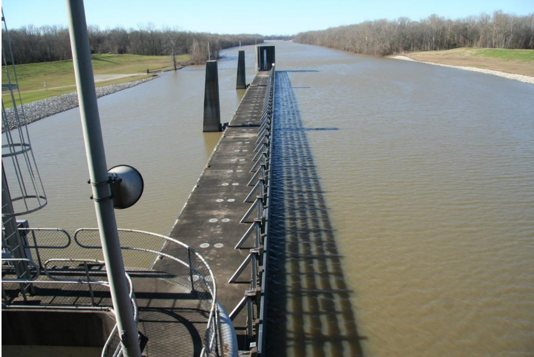
Condition Photo 12: Looking northwest at approach to lock.
