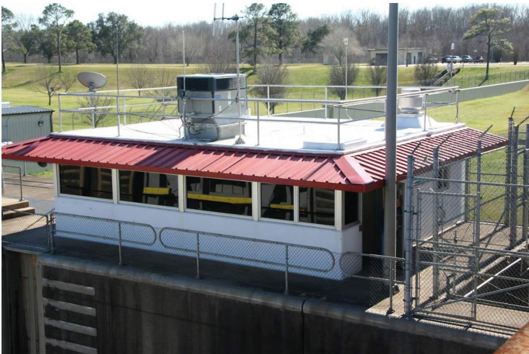
Condition Photo 13: Operator's house as viewed from the lift span deck.
