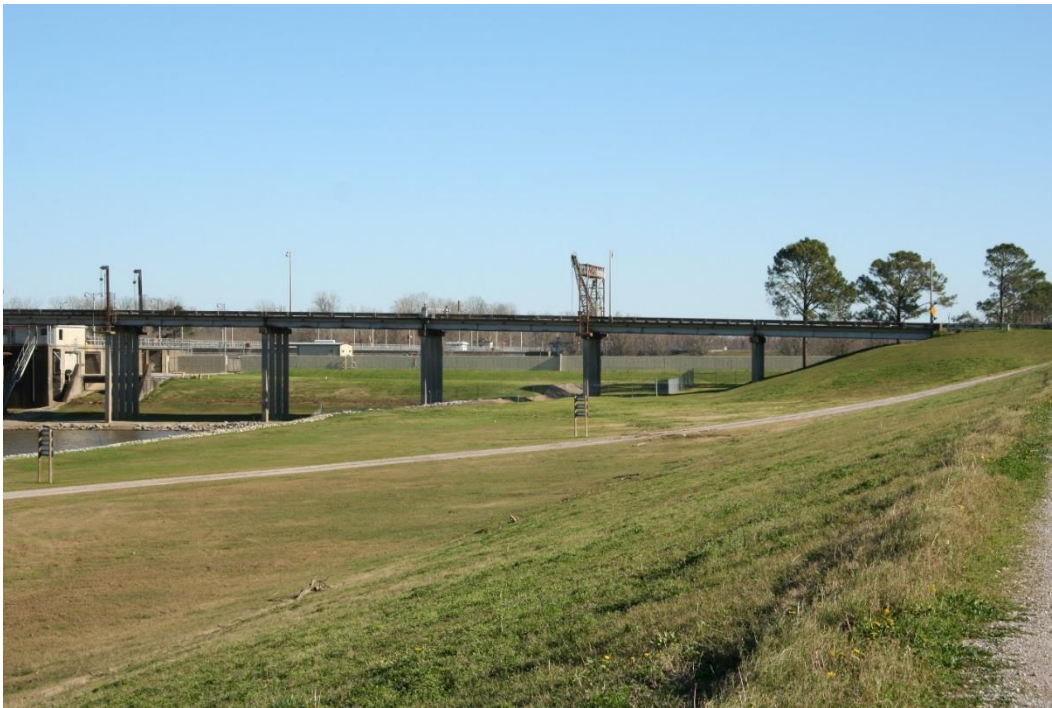
Condition Photo 17: South approach spans, looking southeast.
